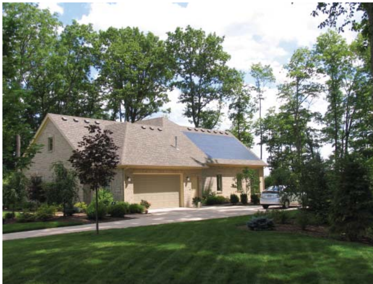
Rob and Linda’s unique home with integrated shingles incorporating flexible triple-junction a-Si:H and a-SiGe:H PV materials on stainless steel foil. A stack of three thin film solar cells, each with different bandgap, enables light collection over a broader range of solar wavelengths than possible with a single semiconductor. This home generates its own electricity from sunlight.
